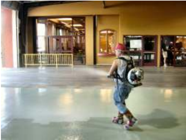
The sand machine in action. Always sand to rejection ensuring full and complete coverage of sand. Leave NO bare spots.
