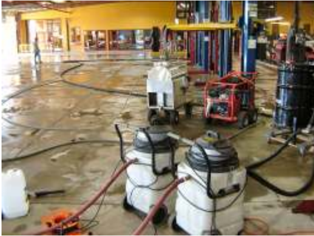
The ORS equipment set-up. Left background is the water heater and blaster; to the right of those is the particle separator with the two vacuums in the foreground.
