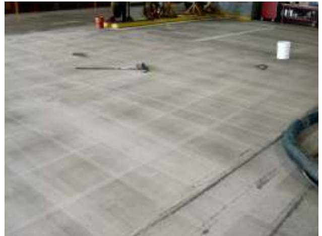
Another shot of the shotblasted deck just prior to the start of the ORS treatment. The dark areas are oil coming back to the surface through the open capillaries of the concrete.
