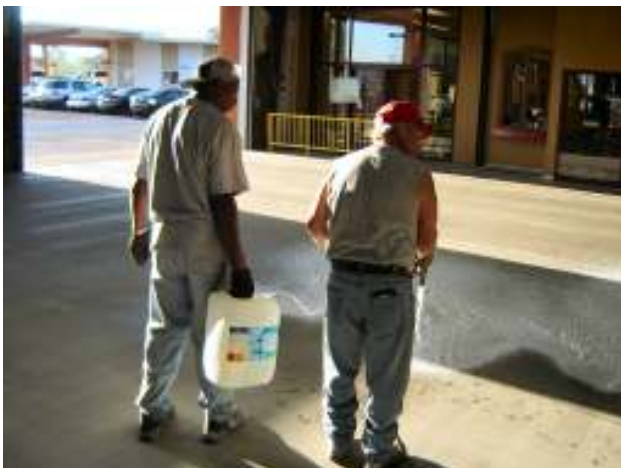
The Petra Coating crew starting the first application of the ORS-D special detergent. The detergent is applied using the Koester foam gun, cold water and ORS-D.
