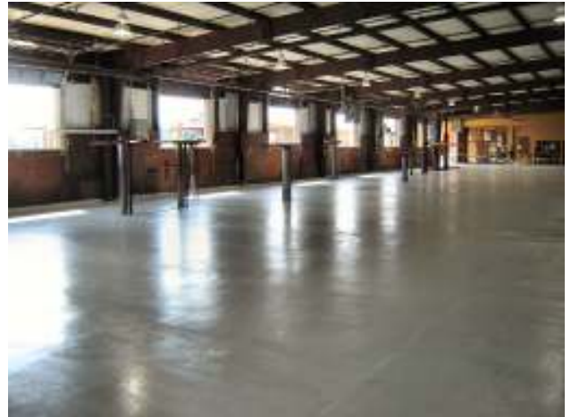
After the floor cures out and is deemed ready for occupancy by the contractor, the Hub City personnel will move all the equipment from the second phase back here to continue working.
