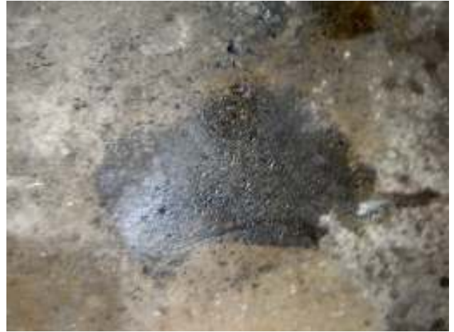
More oil on the concrete. This oil will penetrate deep into the substrate and continually leach back to the surface.
