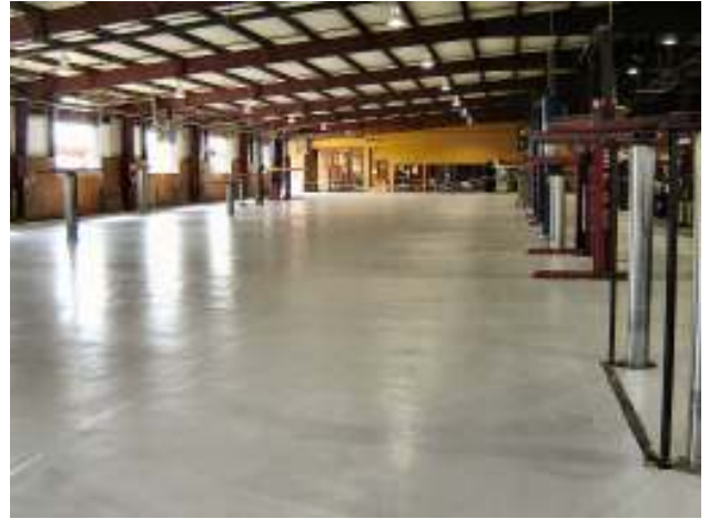
The finished floor looking back toward door A. The floor now has a 10 year Koester warranty against delamination due to oil migration to the surface.
