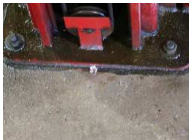
Here is the base of an auto lift leg, note that there is still some oil leaking out from under the leg.
