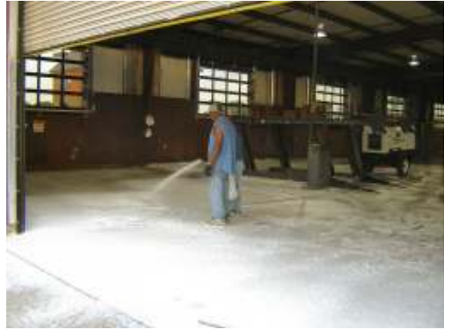
Foaming continues; the second application goes thinner and the spread rate can increase to 350 – 400 sf/gallon (approx).
