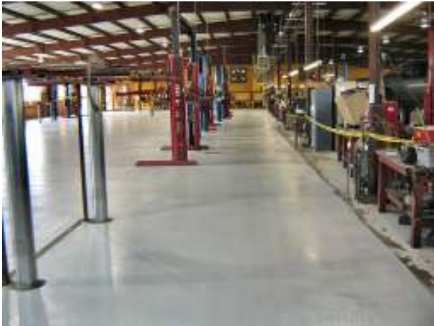
Here is a shot of the finished floor looking down the workbench line. The repair shop on the right was working during the application on the left side.
