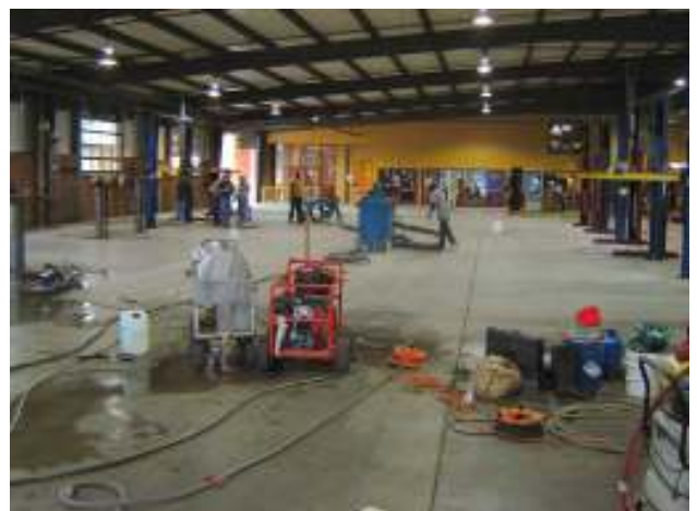
ORS water heater (silver) on left and 5000 psi water blaster on right set up prior to ORS operations. Note shotblasting is still in progress in background.
