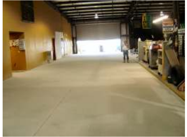
This is the drive through section from door A to door D as noted on the floor plan, the ORS treatment will be applied to the area on the right in photo.
