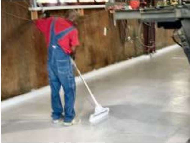
The Petra crew applying the final top coat system of a gray epoxy followed by a gray poly urethane.
