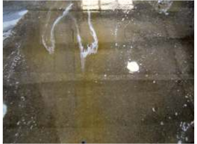
This is a shot of the deck after the hour wait on the foam which has gone from a white color to clear. Note the oil as a yellowish stain in the center.
