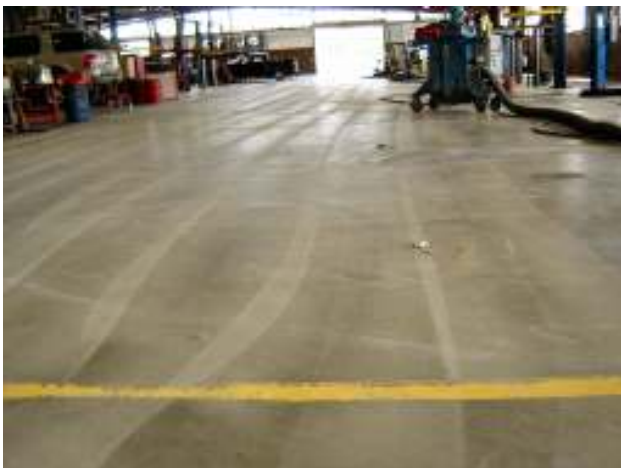
This is a shot of the first phase floor of approx 15,000 sf looking down toward door B. Note the shotblaster on right.
