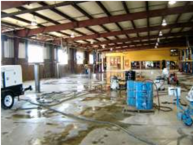
This shot is a little further back from the shot above. Note the two waste water (blue) barrels on the skid with the hoses from the vacuums.
