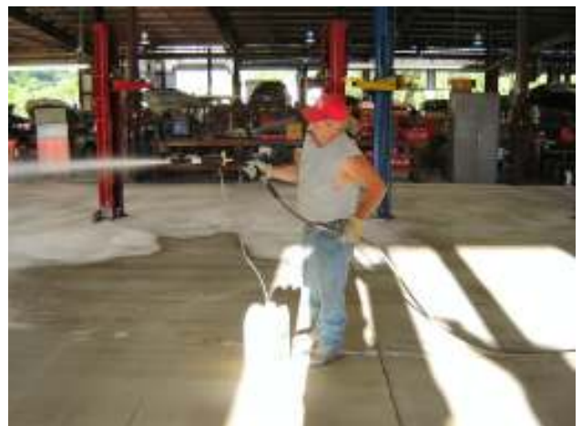
The detergent is mixed at the nozzle along with 5000 psi cold water to form the "foam carpet" that will be allowed to sit for approx 1 hour.
