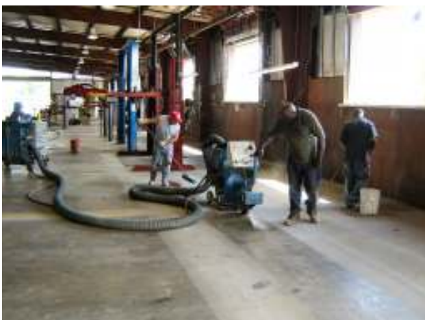
Shotblasting operations in progress. The floor was double shotblasted to remove a surface sealer, old wax, dirt and to profile the floor.
