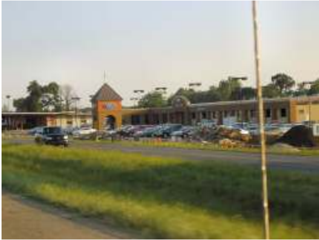
The Hub City repair shop to be treated with the ORS is the building with all the windows on the right above. Door A is on building front just to the right of the tower for reference.
