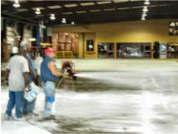
The first area by door A gets the second foaming application. Most floors with this amount of contamination will require two applications of the ORS-D.
