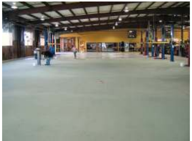
The ORS process is continuing behind the camera, in front all coated and sanded with 12 hour cure. Note in the far background the crew is applying the final top coat to the first section.
