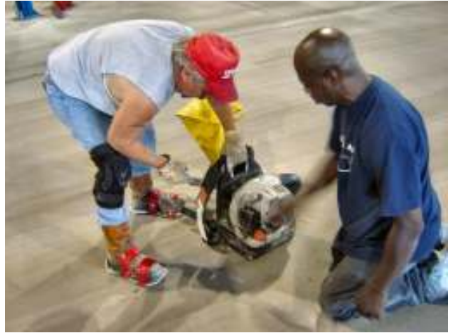
Petra Coatings crew enlists the aid of a sanding machine consisting of a blower and a sand hopper (yellow) for even sand distribution over a large area.
