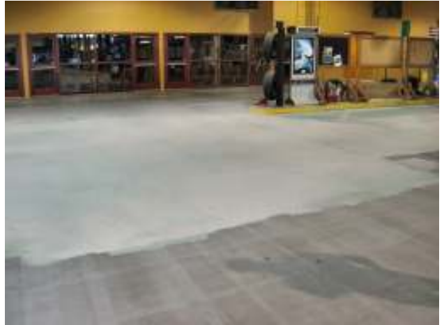
The first section cleaned, coated and sanded. Allow a 12 hour cure before excess sand is swept up. The crew gets some rest.
