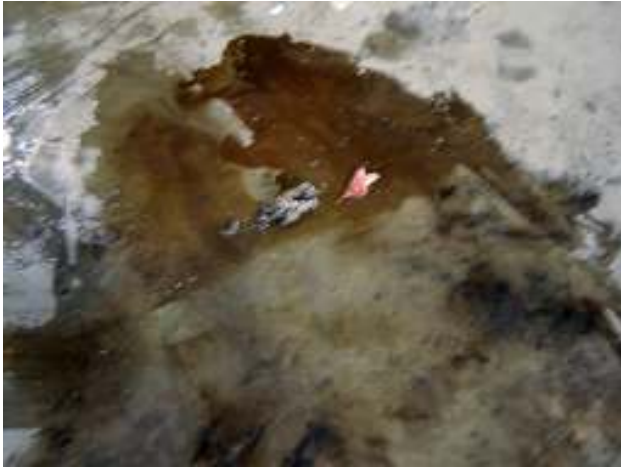
This slab is oil contaminated. Here oil is puddle on the surface by one of the lifts.
