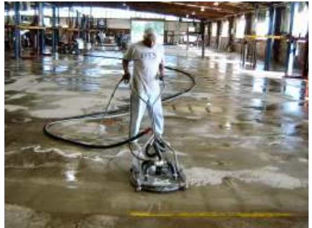
Second application spinning operations are also stepped up and a much faster floor speed can be used.
