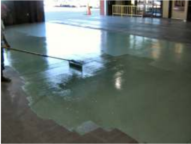
Finishing up the first section of coating. Note the change in color of the material toward the top of the paint area as the surface starts to set up-time to sand.
