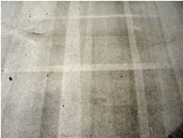
Here is a shot of the aggressive double shotblast pattern. Note the 90° pattern and the oil (dark areas) coming back up.
