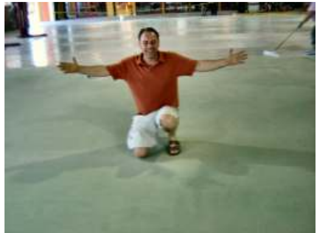
Joachim Bohlmann, ORS Manager of Koester American signals all is well with the ORS application. The crew continues its application of the top coat in the background.
