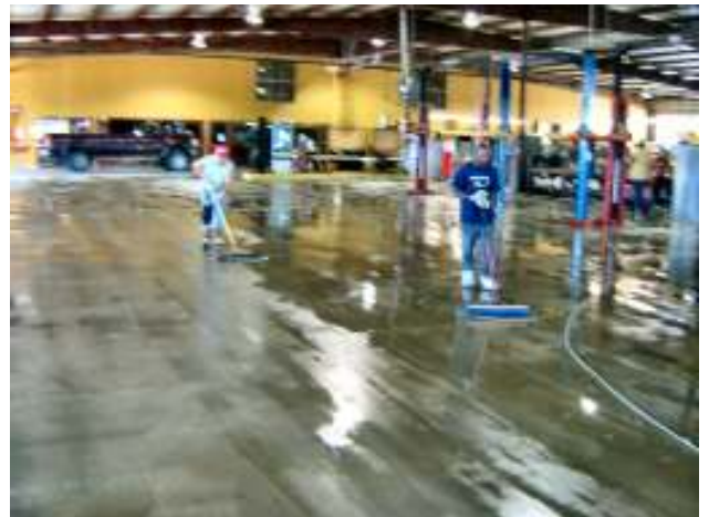
After spinning operations, the crew tends to waste water management and removes all excess water.
